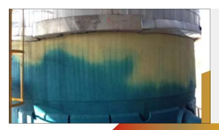
CT-IP180 is a one time warning system. The colour change is permanent.
